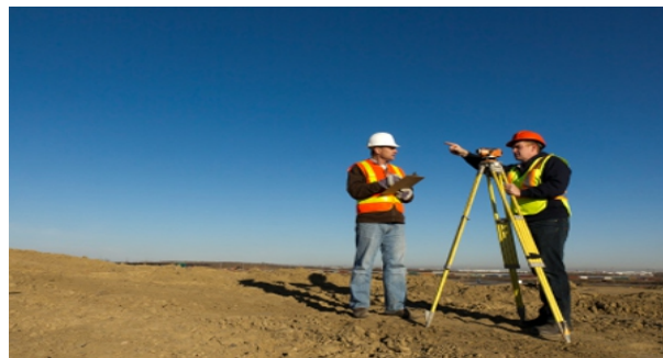
Site Surveying and soil testing.
