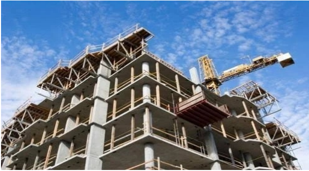
Civil construction with Services (Electrical, HVAC, Plumbing and Fire Fighting)
