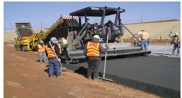
Road construction and Street Beautification
